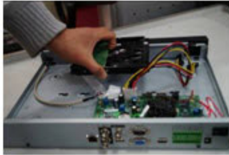
Figure B-3 Placing the HDD
